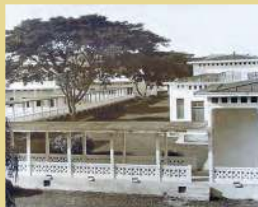
Walkways inside the hospital compound
